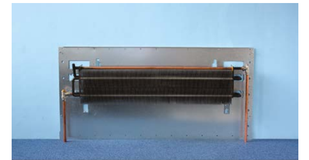
Emitters and valves (1st fix)
